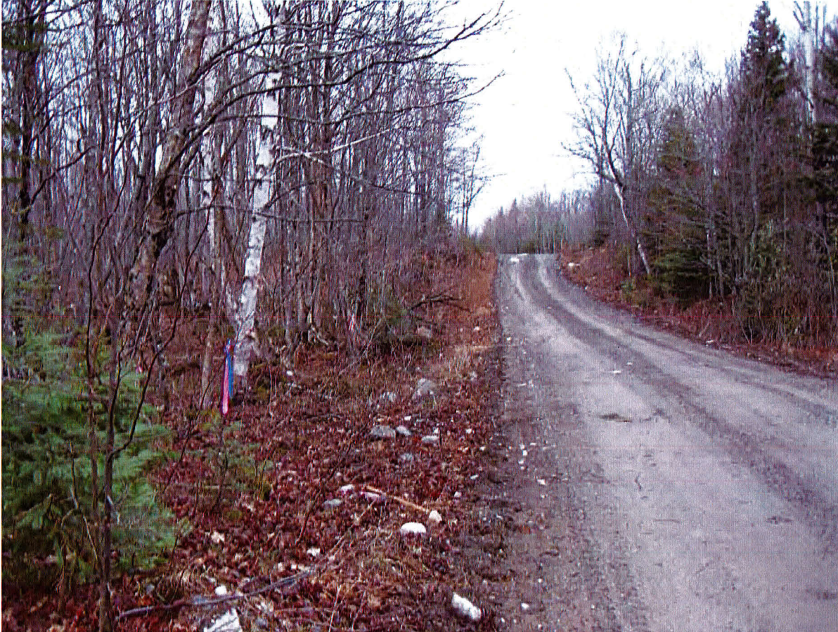
Attachment 9: Photo Along CR 595 Alignment
